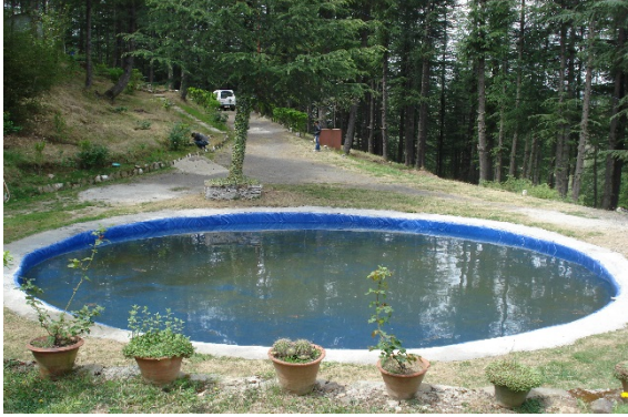
Water Storage Tank
